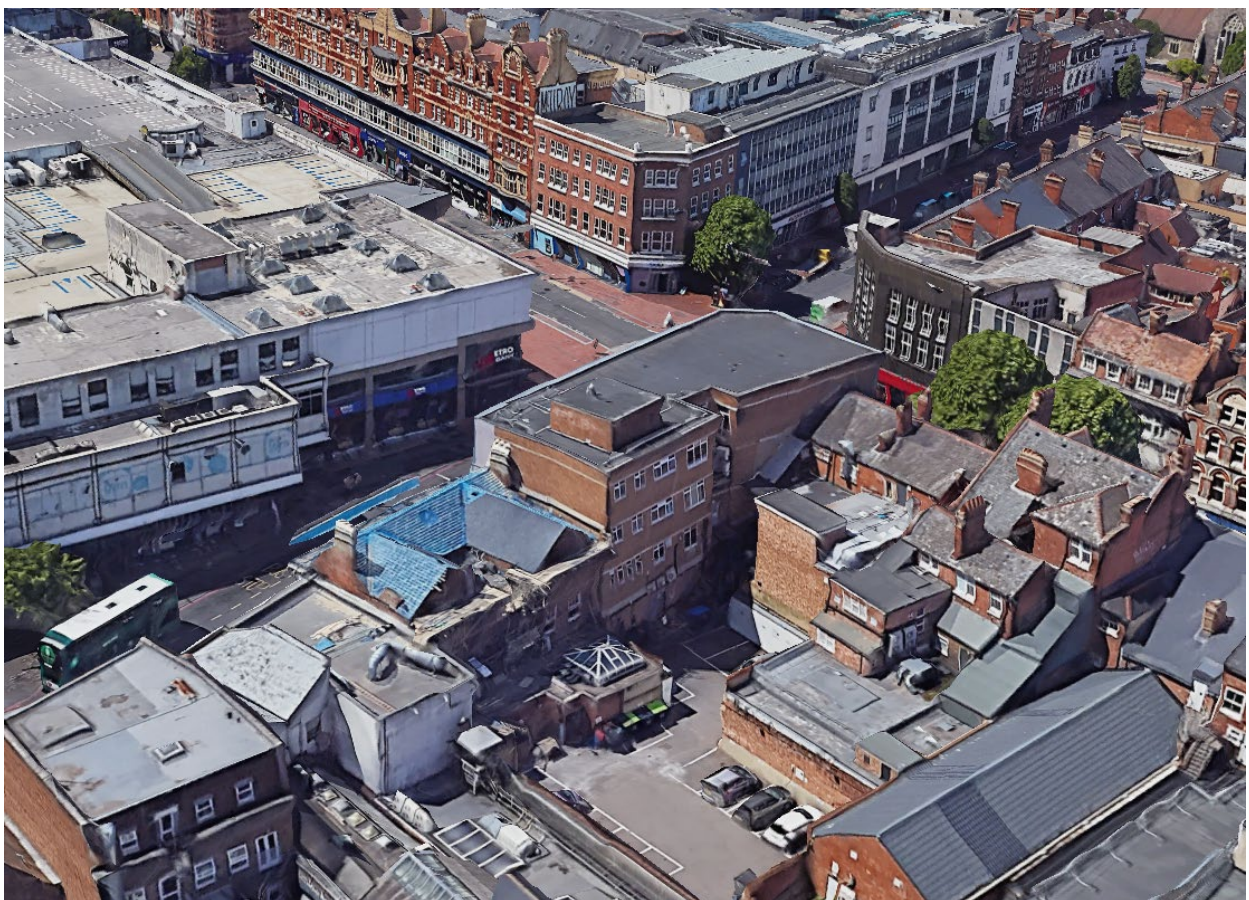
Google Maps aerial viewpoint from the south-east, showing the rear elevation and parking area
