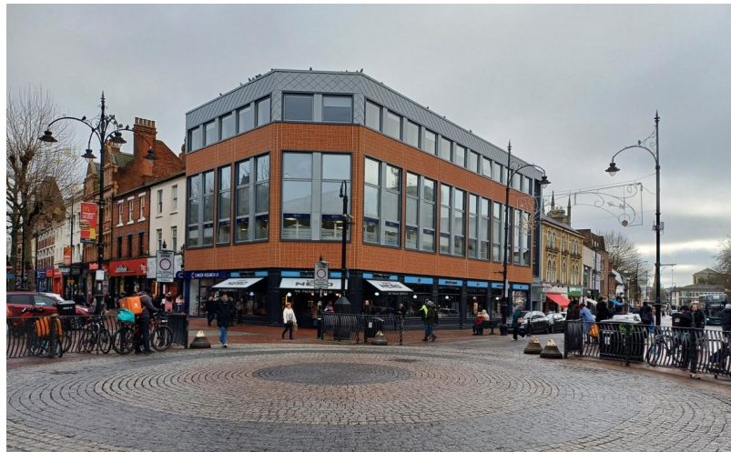
Figure 2 – Present view showing both the Broad St & St Mary's Butts frontages
