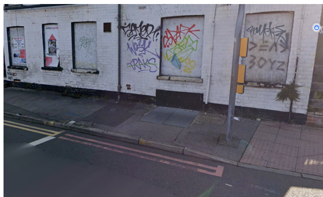
Figure 15 - Cellar door on Bedford Road frontage
