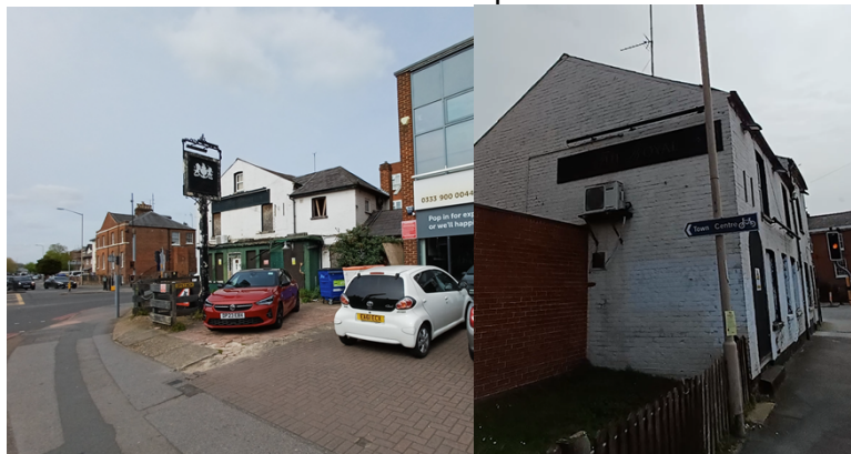
Figure 2 - Site photos (10 April 2026)
